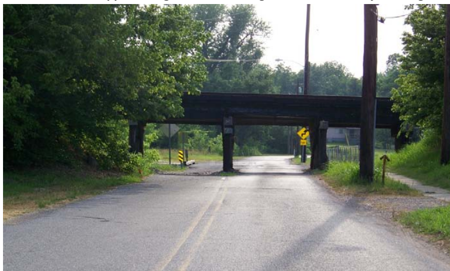
Exhibit 8: KY-1826 continued approach to Railroad Bridge and Project Bridge looking west
