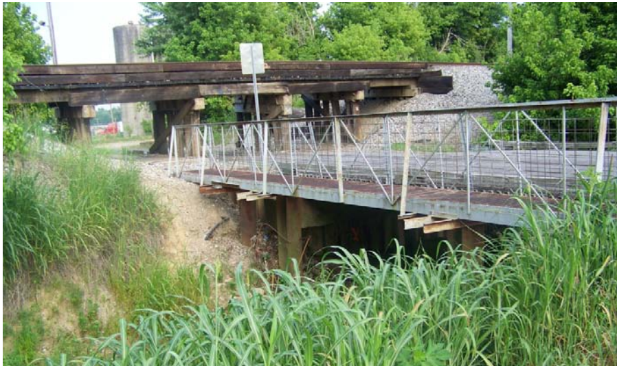
Exhibit 10: KY-1826 Pedestrian Bridge looking south west from north east
