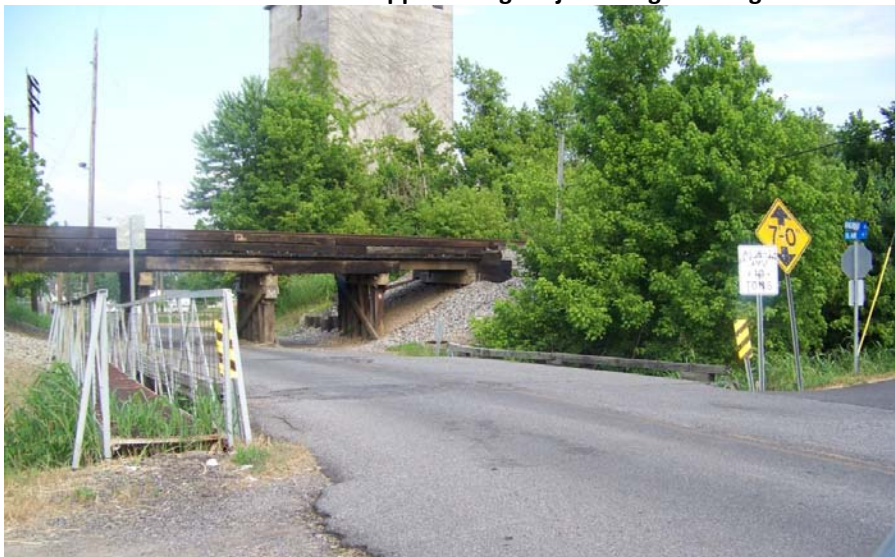
Exhibit 7: KY-1826 approaching Pedestrian Bridge connected to Project Bridge looking east
