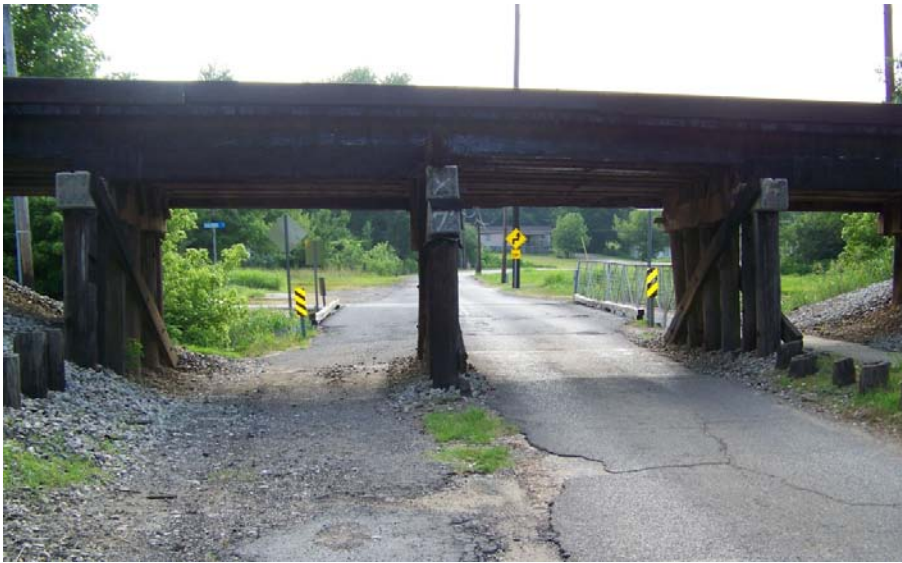
Exhibit 9: KY-1826 gazing through Railroad bridge to Project Bridge looking west
